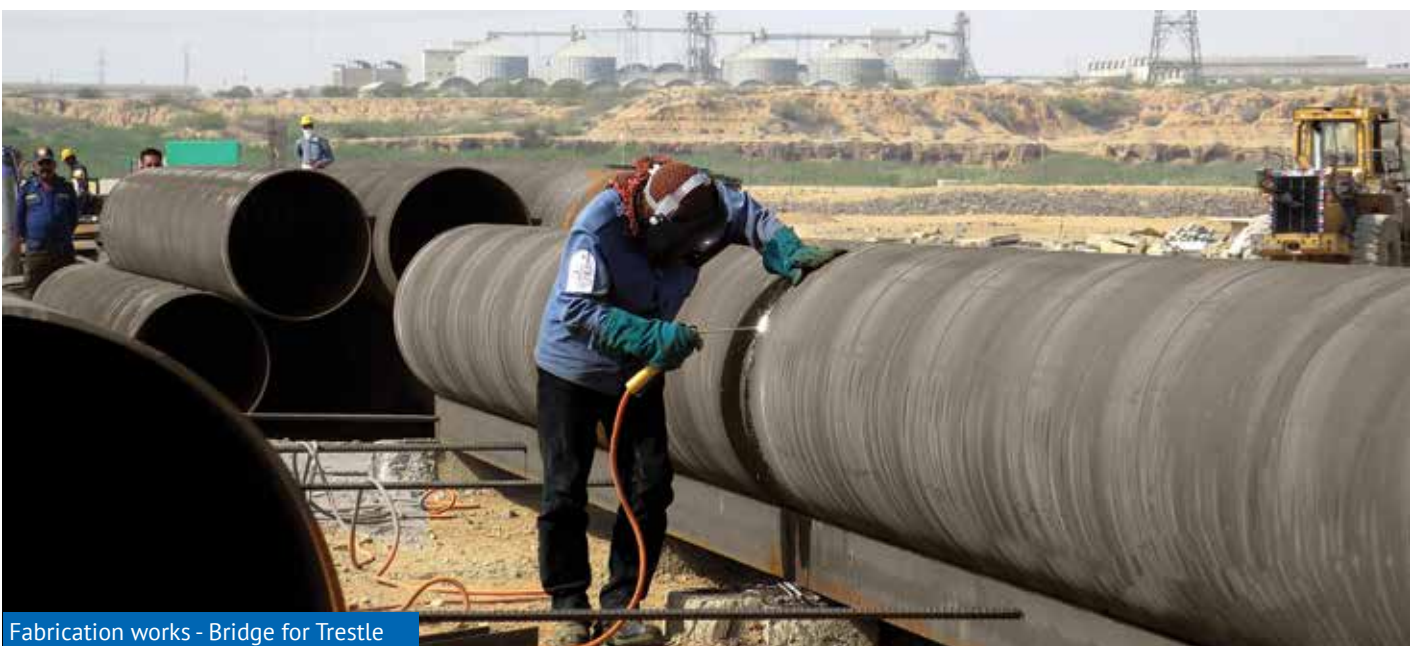
Fabrication works - Bridge for Trestle
