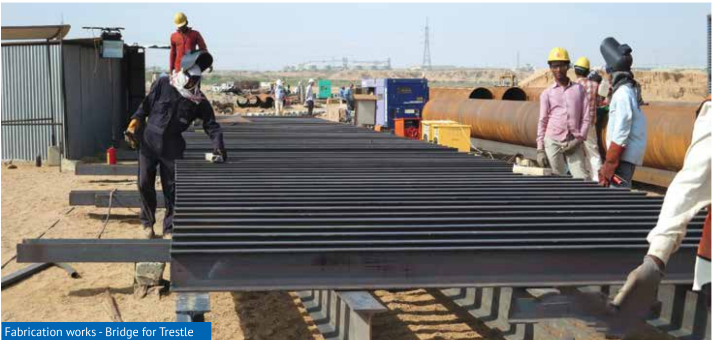
Fabrication works - Bridge for Trestle
